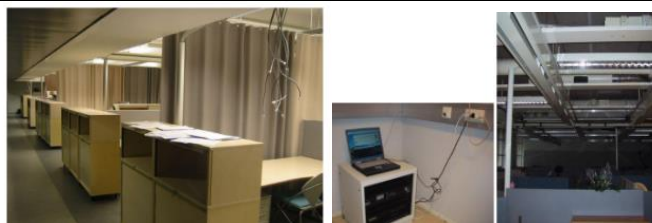
Fig 3a & 3b: a) Office 3 when curtain are shut b) Sound masking central unit and one of the black loudspeakers installed above electric shelf
